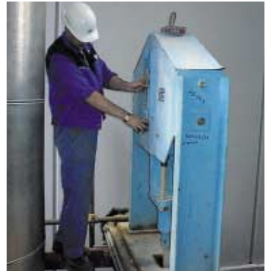
Checking piping movements
