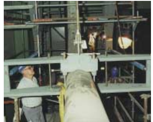
Supervision of support installation
